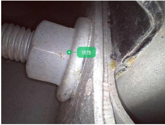
右前纵梁:锈蚀
